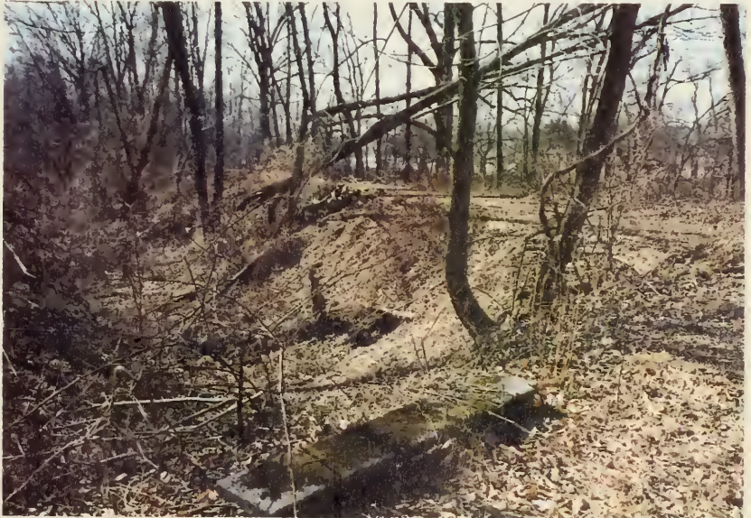
Fig 110 The overgrown path of the old train line near the mill at Anselma. Photograph by the author 1995.
